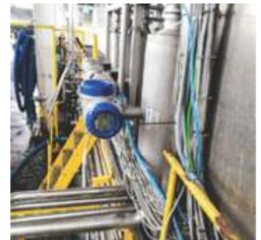
Flow measurement at raw milk reception with the OPTIMASS 1400
